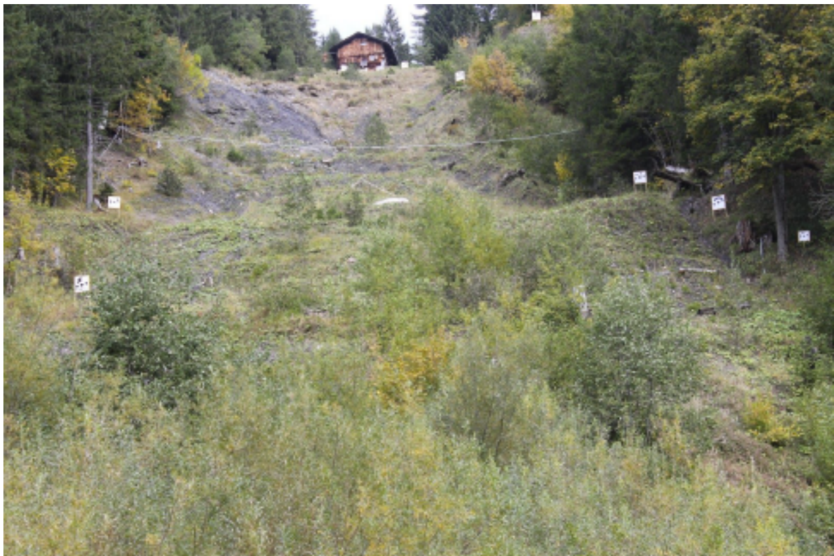
Photo from one of the cameras showing the landslide. Some targets can be seen (white squares with black markings)
