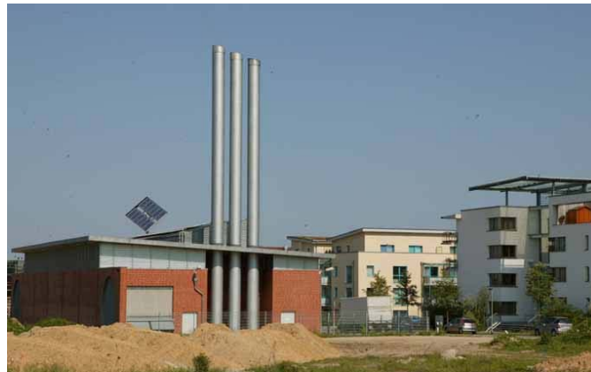
Figure 11 Decentral cogeneration plant
