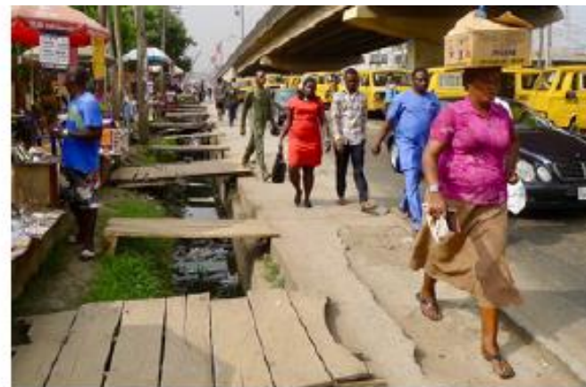
Risky open drains
