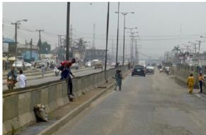
Lack of pedestrian crossings
