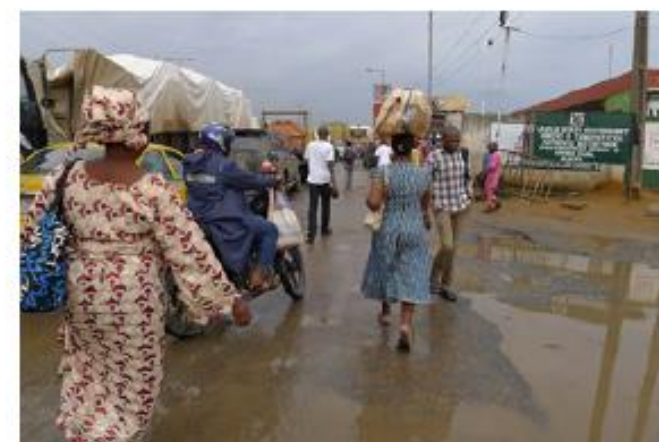
Lack of storm water drainage
